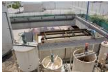
Water and oil separation plant
